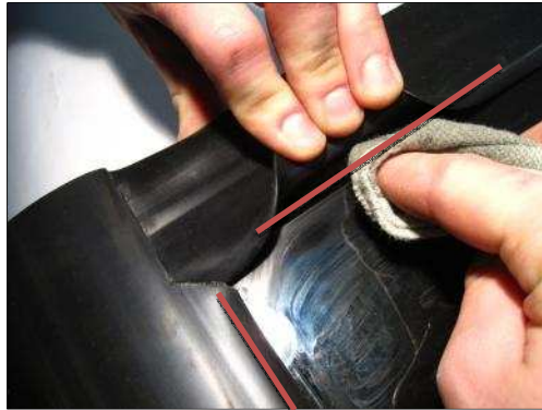
Cleaning before sealing
