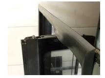
8.3.2. Cut a small "V" shaped piece out of the rubber (on the topside of the door).
